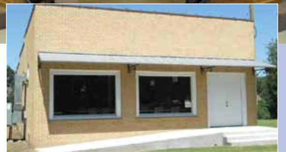
Renovations at a former grocery store, located on Hwy. 77, are now complete and the building is ready for use as Rosedale's Community Center.
